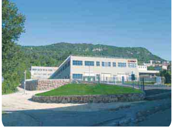
Aignep new plant, with a covered surface of 12.000 m 2 .
